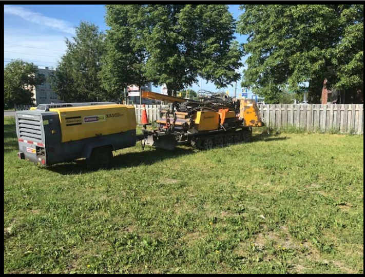
Drill Setting Up at MW1 – June 19, 2020
