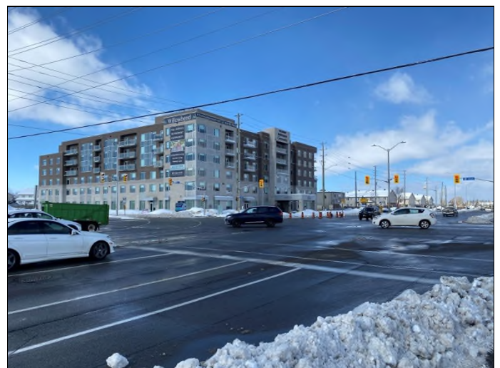
6. 1980 Trim Road – Willowbend Retirement Community building located to the northwest of the Site.
