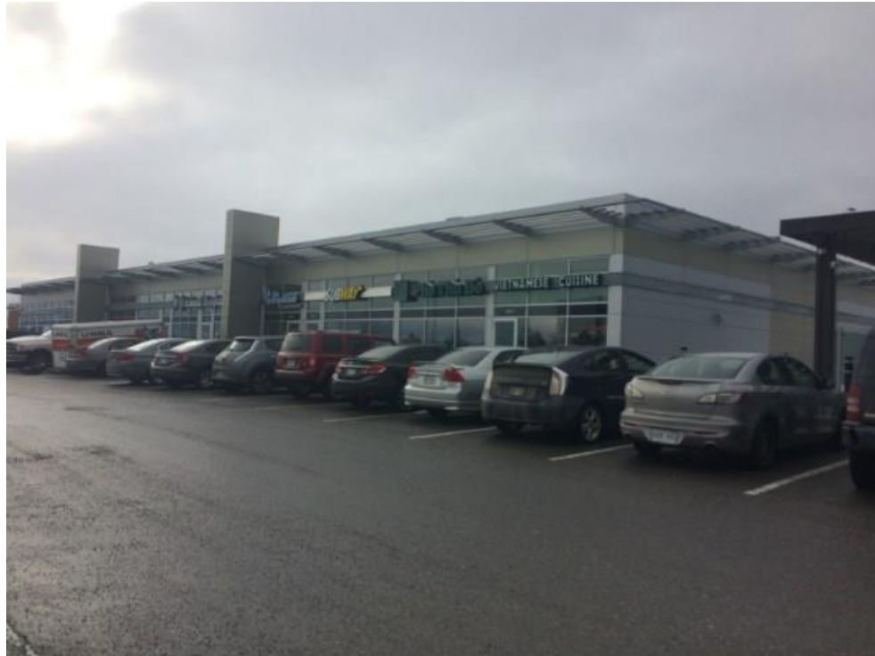
Photo 7: Photo of a commercial plaza located on the surrounding lands southwest of the Site.
