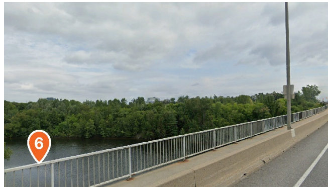
Figure 13: Looking northeast toward the site from the Michael J. E. Sheflin Bridge
