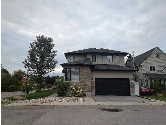
319 Spencer Street, viewed from Spencer Street
