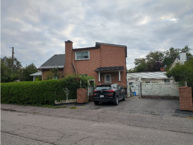
323 Oakdale Avenue, viewed from Rockhurst Road
