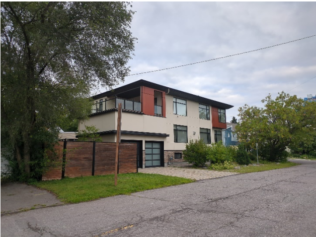
53 Gould Street, viewed from Rockhurst Road
