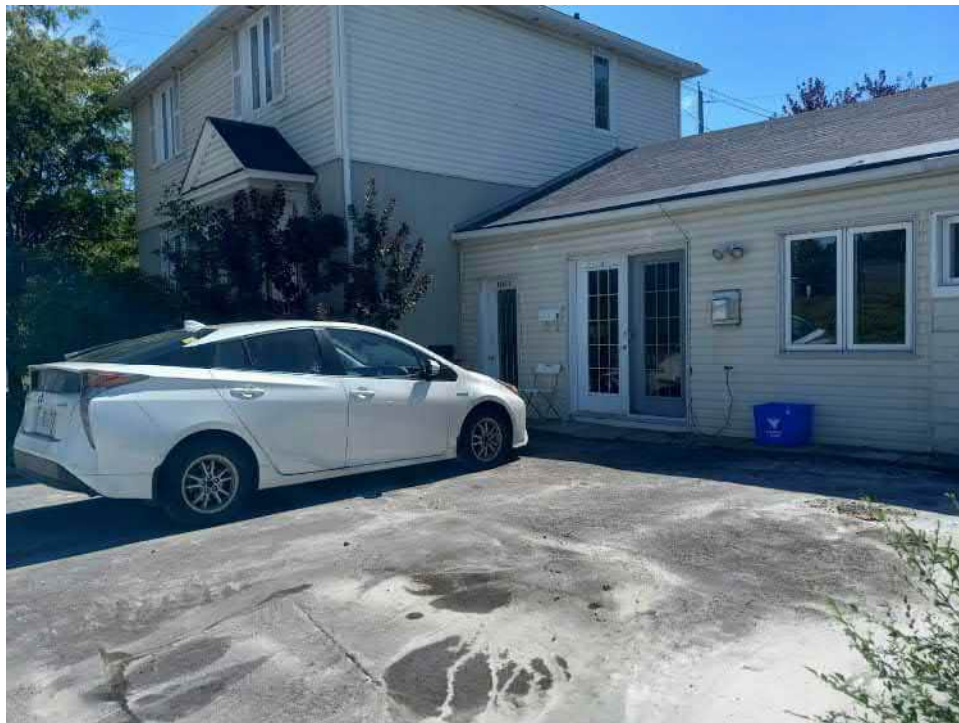
Photo 2: View of the front entrance and entry into a residential unit. Minor staining observed on parking lot.
