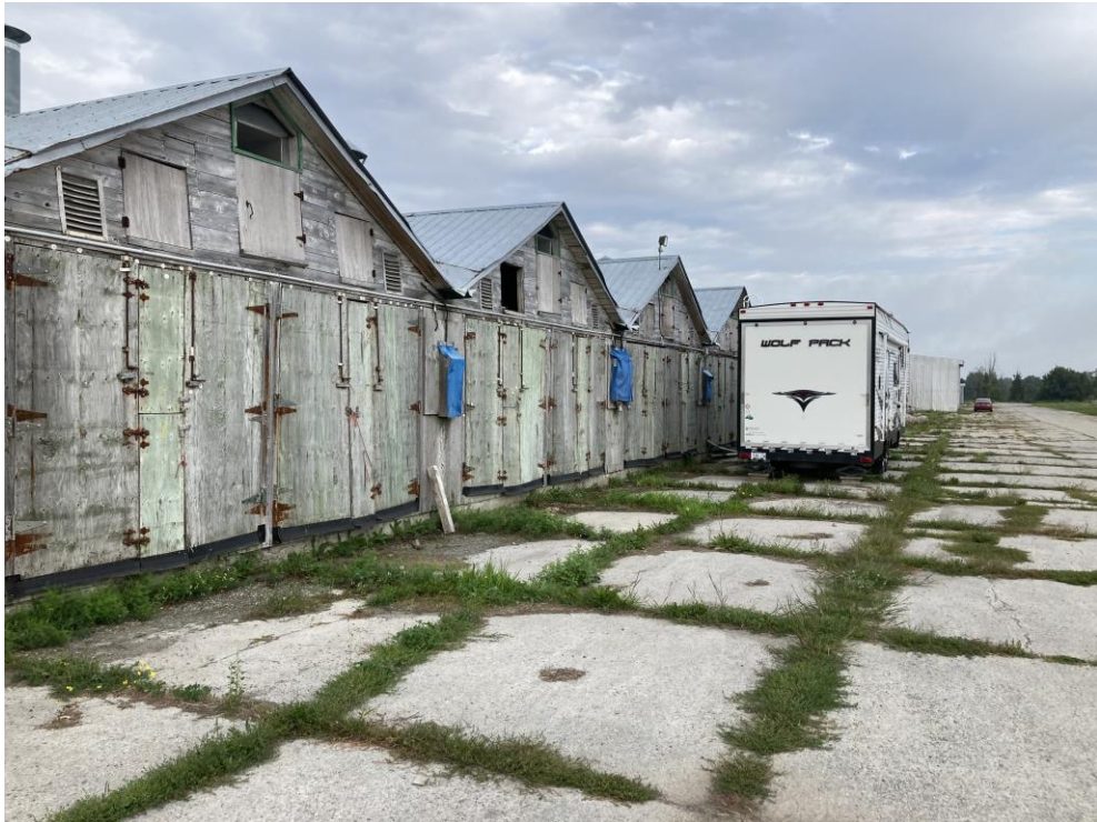
Photo 5. View of mushroom facility buildings and openings in eaves.
