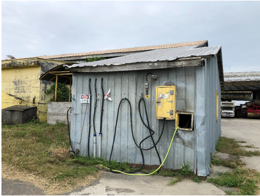
Photo 5 - View of building that houses drilled water well TW-2.
