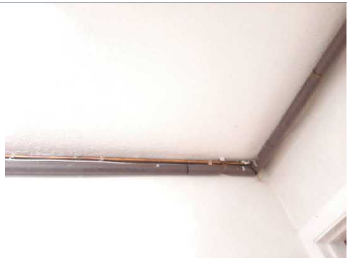
Picture 3 – Piping inside site building
