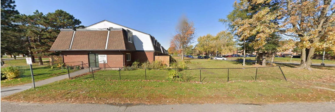
Figure 13. Surrounding Built Form: Low-rise Residential North of the Site at 1958 Jasmine Crescent (Looking Northwest)
