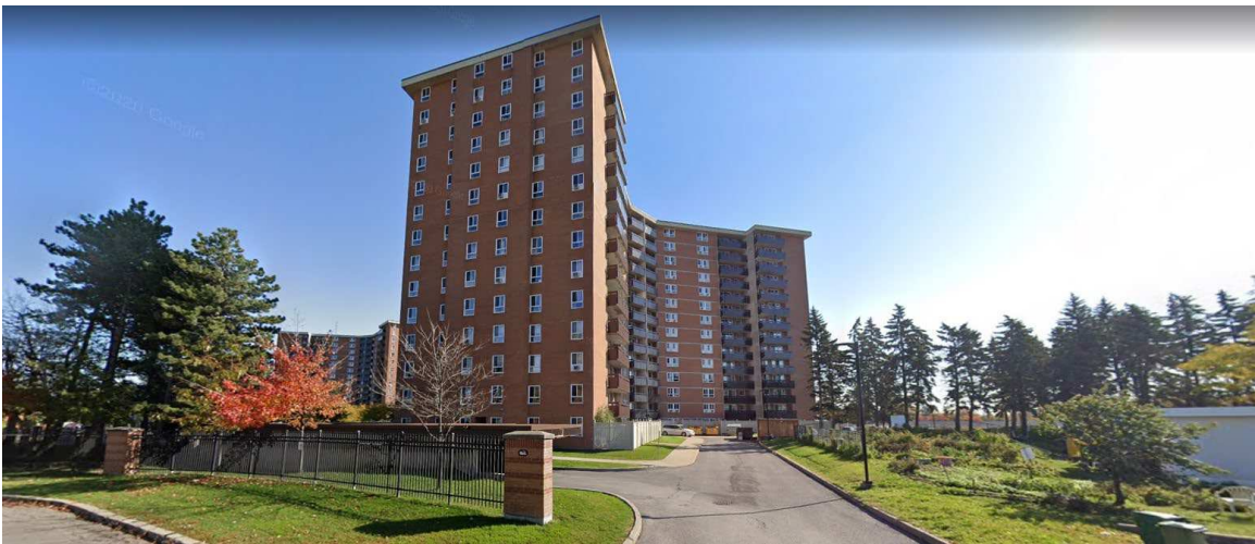
Figure 9. Surrounding Built Form: High-rise Residential East of the Site at 2000 Jasmine Crescent (Looking East)
