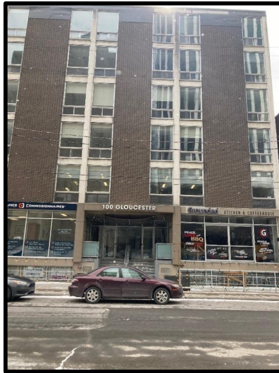
Photograph 1: Street view of 100 Gloucester Street, looking south.
