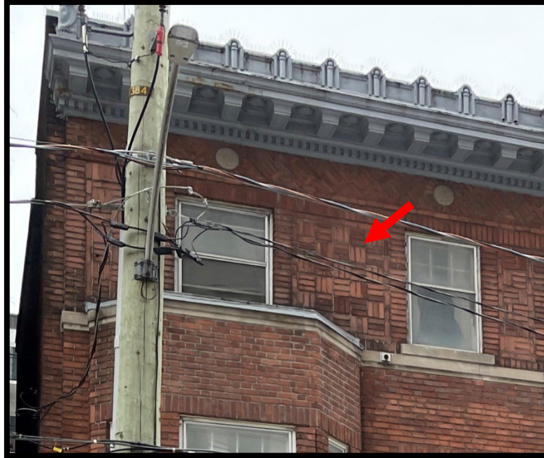
Figure 15: After the Wendell Apartments block was remodelled in 1941, the original facade disappeared behind an addition that likely contained a fire-resistant staircase. The remodelling reinstated or replaced the decorative cornice, but obscured and removed elements that contributed to a more recognizable Italianate style. One of these elements as the basket-weave brickwork (arrow). Source: Matrix Heritage, 2023.
