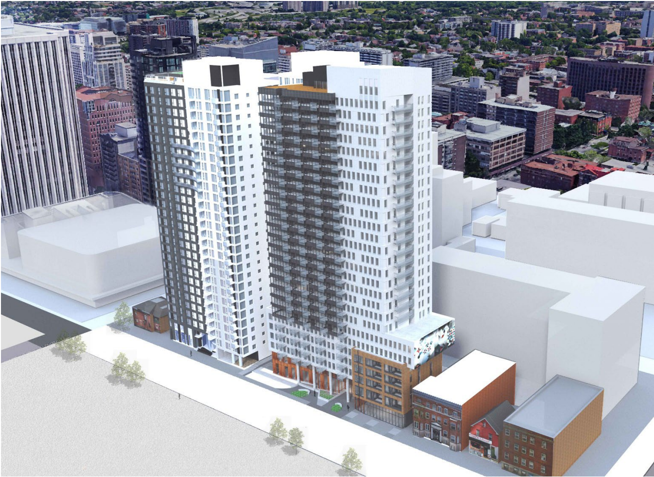
Figure 4 Aerial View looking south-east.
