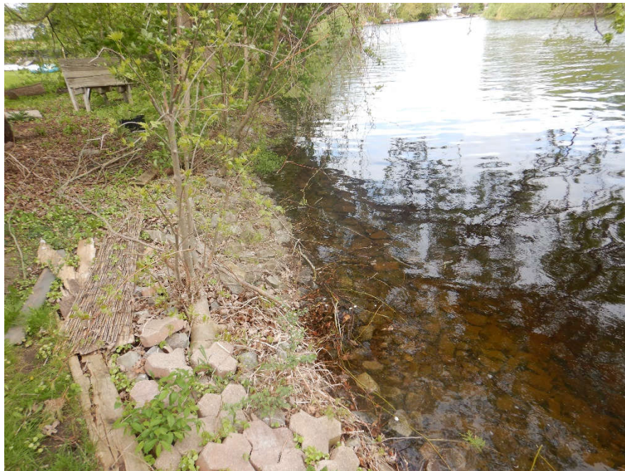
Photograph taken facing downstream, bank materials extended approximately 1-3 m into the water, and 1-2 m up the channel banks.
