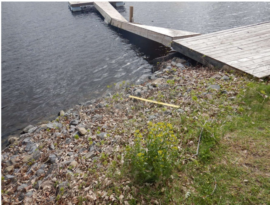
Photograph taken facing upstream at the upstream extent of the subject lands. A majority of the shoreline was composed of rip rap. Private docks were present at the shoreline of most residences.
