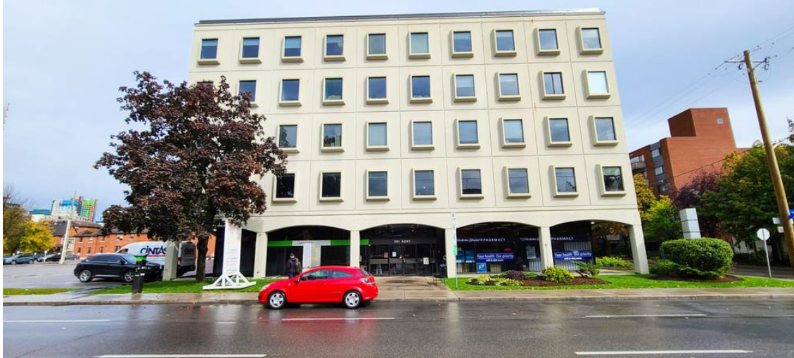
Figure 11: The view from Kent Street presents a façade identical to the other three sides with an arched arcade and the ground floor retail set back. The upper floors are a cream toned concrete with score lines defining each level and evenly spaced punched windows set-in a raised frame. Source: Google maps.
