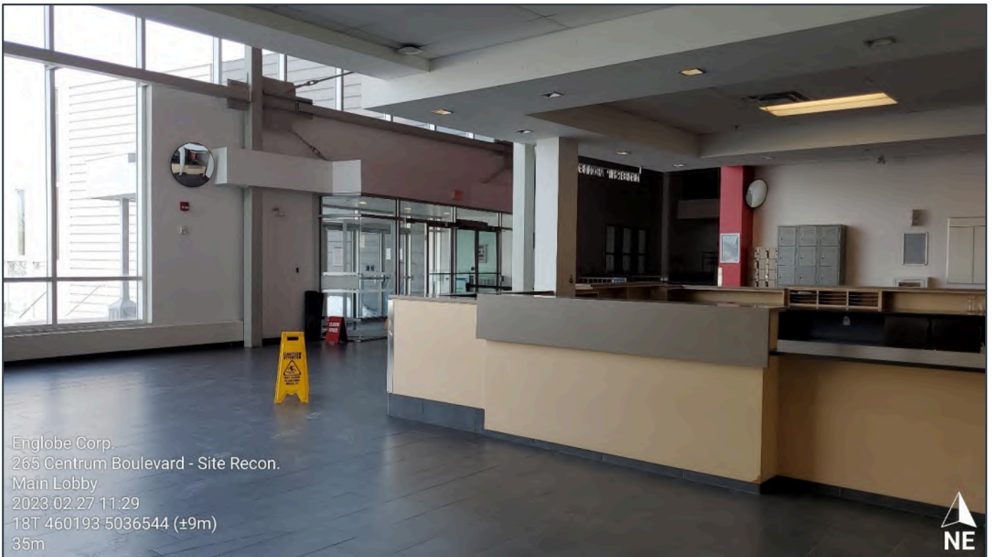
Site Photograph 10: Overview of the front lobby area.
