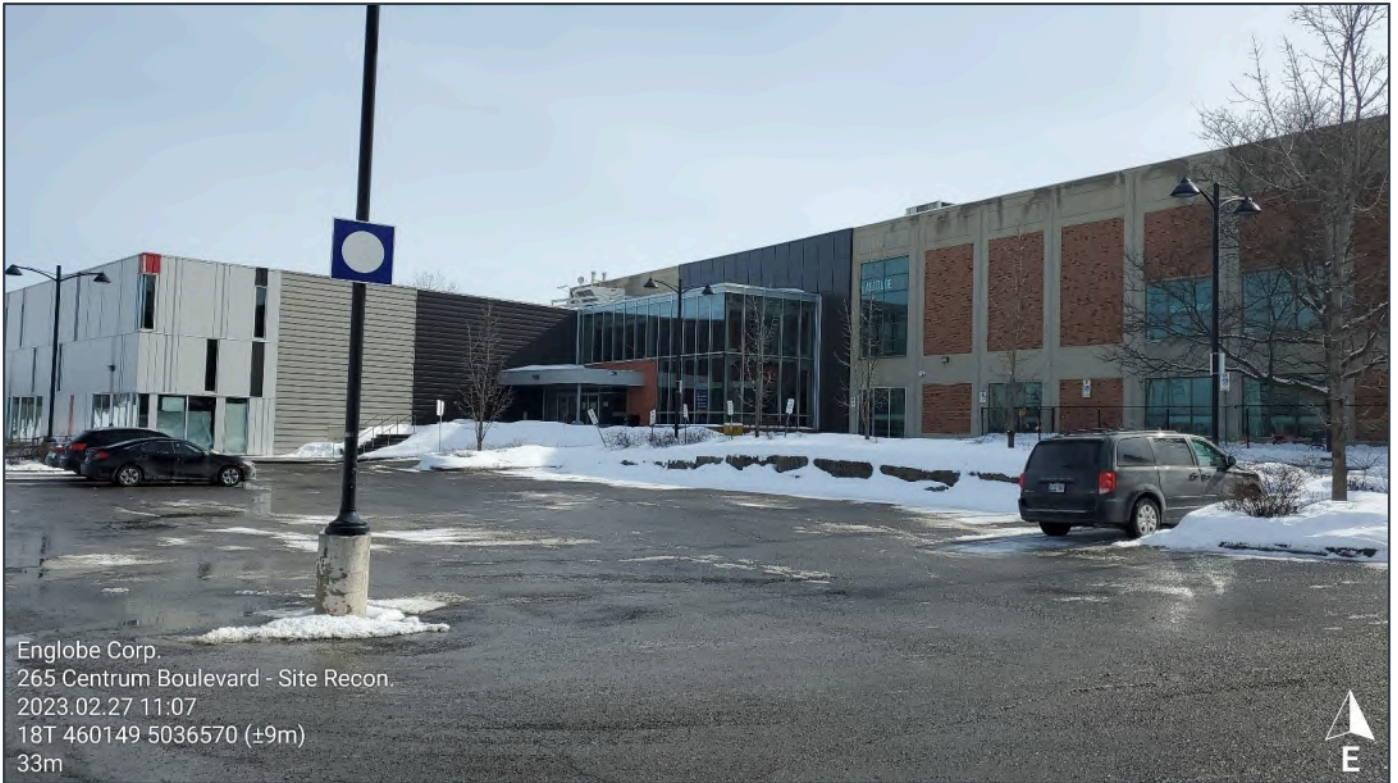
Site Photograph 1: Overview of the Entrance to the Site building (original build and new addition).
