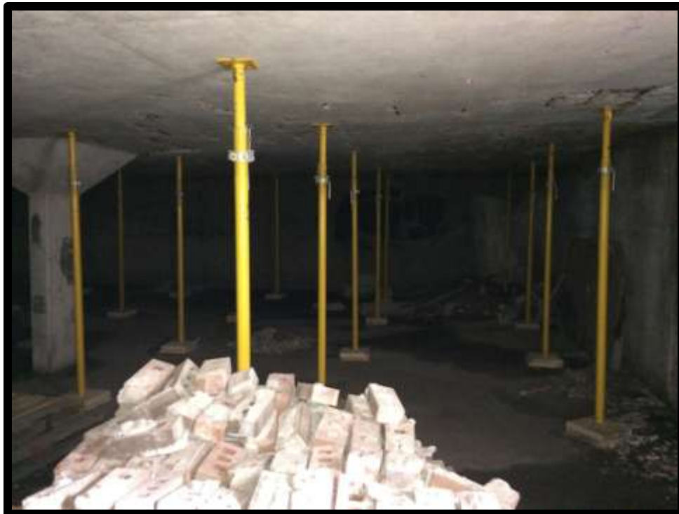
Photograph 2: View of interior of lower portion of the parking structure, facing east from the western portion of the structure. Some debris and bricks are present in the foreground.
