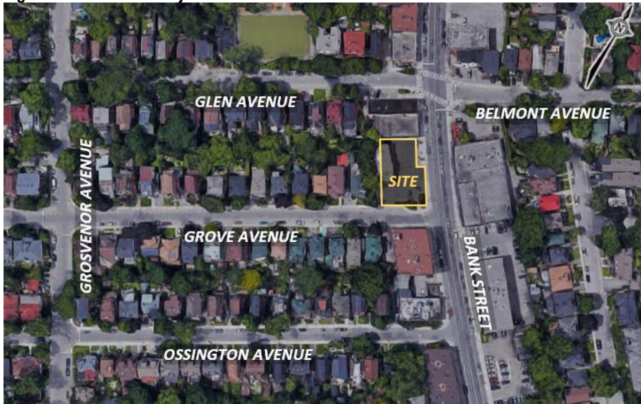
Figure 1: View of the Subject Site
