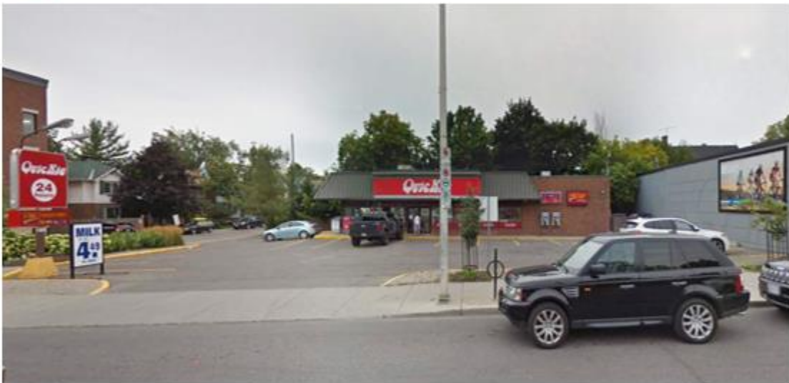
6 BANK ST VIEW TOWARDS PROPERTY – WEST
