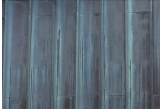
Figure 22. Standing seam copper roofing (ERA, 2021).
