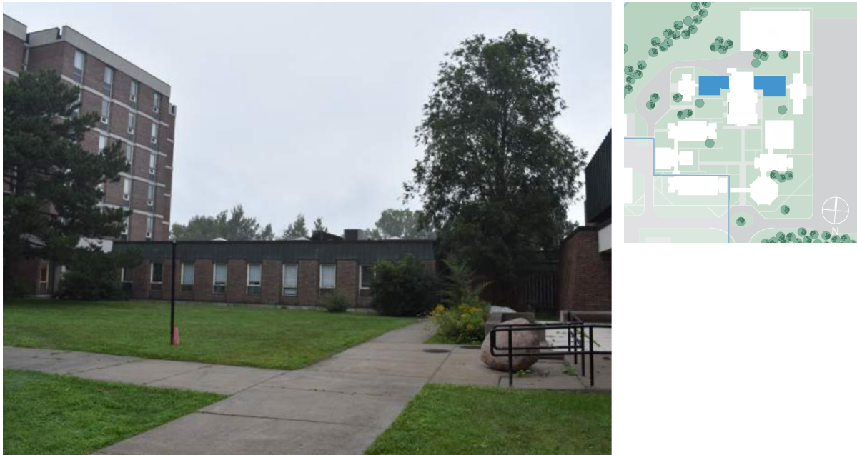
Figure 3. Building B, from Sisters' courtyard (ERA, 2021).
