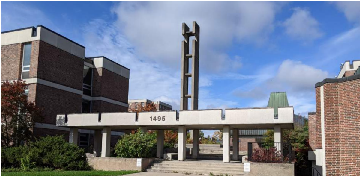
Figure 12. Main entrance canopy, with Campanile behind (ERA, 2021).
