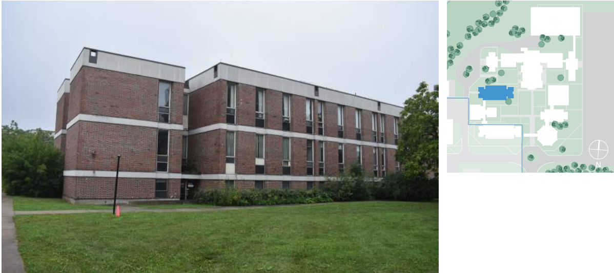
Figure 9. Building J, from Sisters' courtyard (ERA, 2021).
