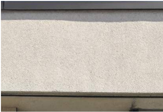
Figure 23. Aggregate-faced concrete paneling (ERA, 2021).
