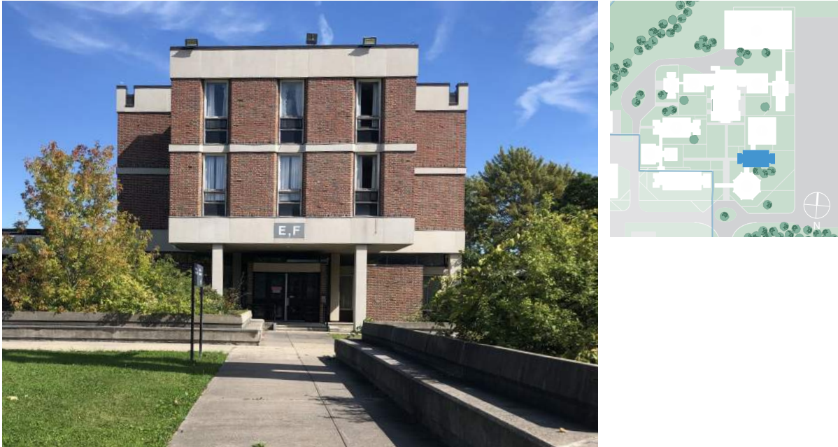
Figure 6. Building E, west elevation (ERA, 2021).
