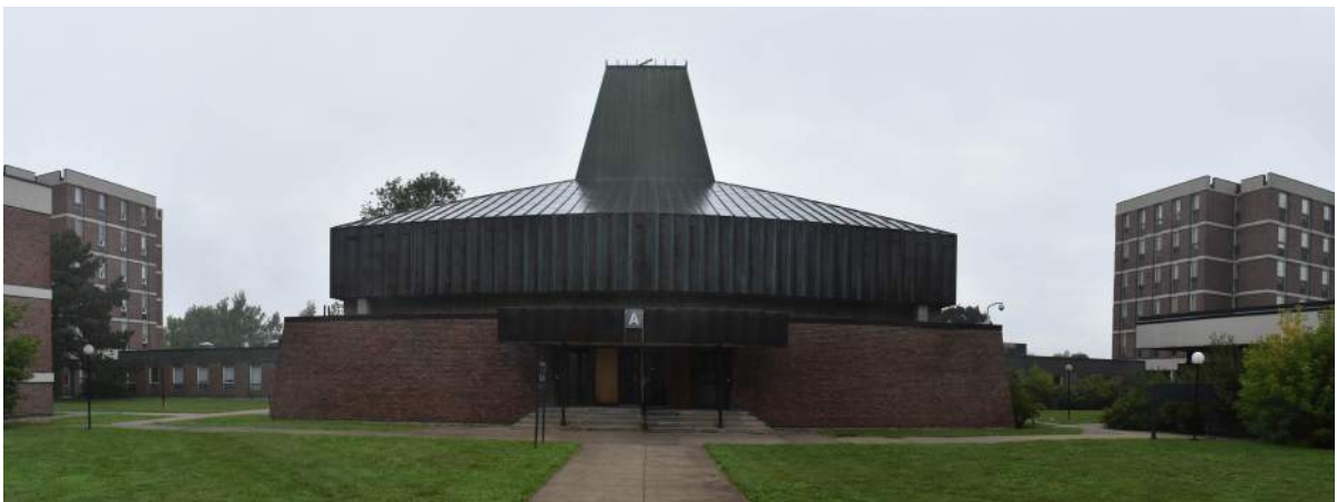
Figure 30. The central academic courtyard, facing north. Image focuses on Building A, but the Sisters' (left) and Novitiate (right) Courtyards can be glimpsed on either side (ERA, 2021).
