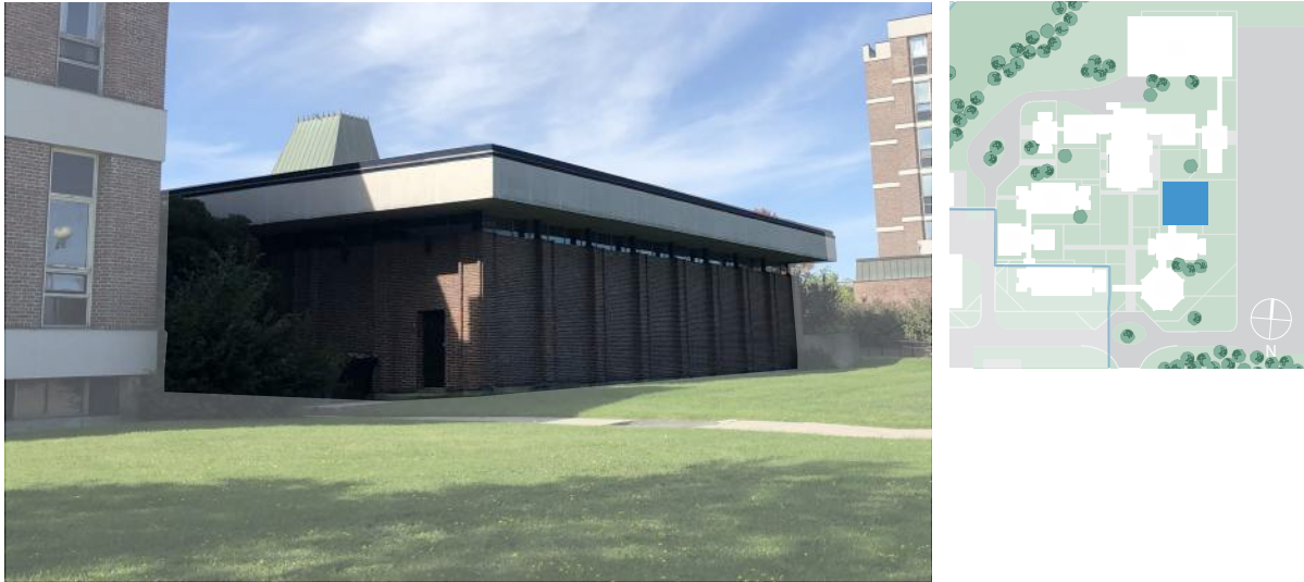
Figure 5. Building D, viewed from southeast (ERA, 2021).
