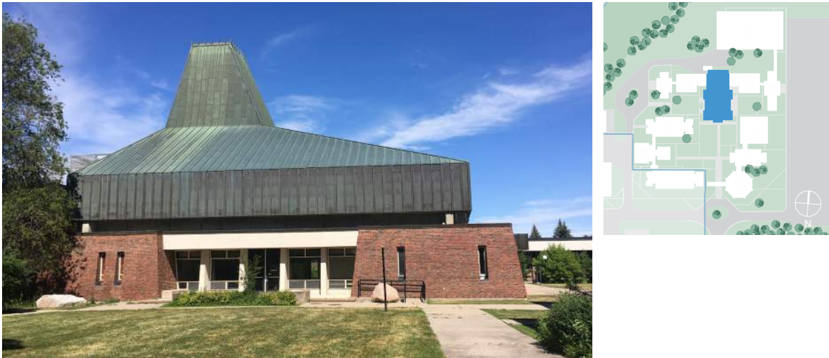
Figure 2. Building A, west elevation (ERA, 2021).
