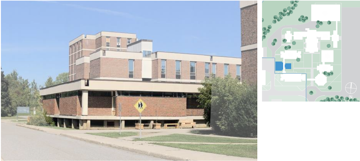
Figure 8. Building I viewed from southwest (ERA, 2021).
