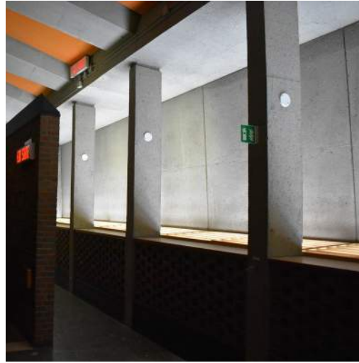
Figure 18. Building A, columns and water detail (ERA, 2021).
