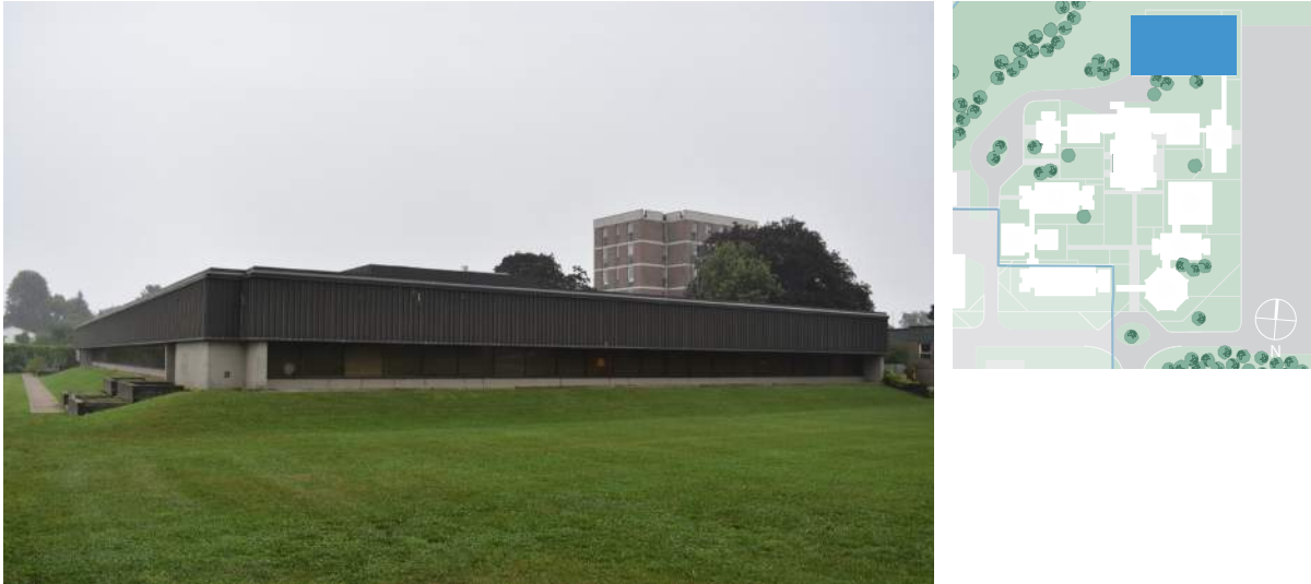
Figure 10. Building M, west elevation (ERA, 2021).
