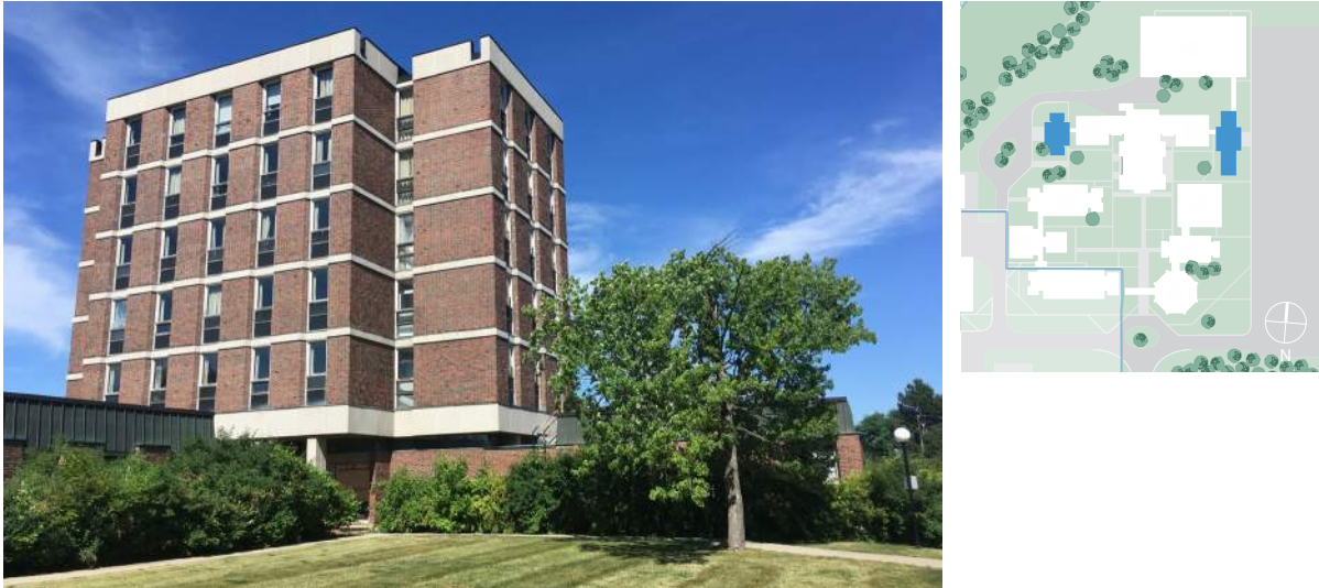
Figure 4. Building C, from novitiate courtyard (ERA, 2021).
