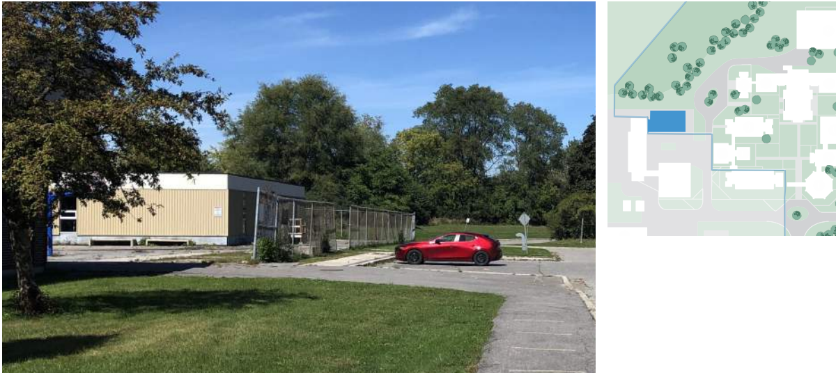
Figure 11. Building N, viewed from south-east (ERA, 2021).
