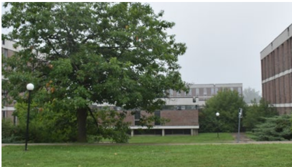
Building H, east elevation
