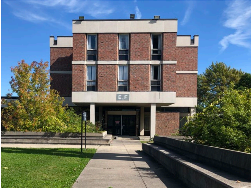
Figure 18. Building E, west elevation (ERA, 2021).
