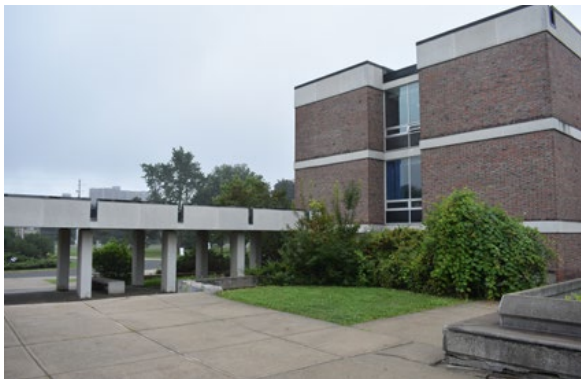
Figure 32. Existing conditions at main entrance (ERA, 2021).
