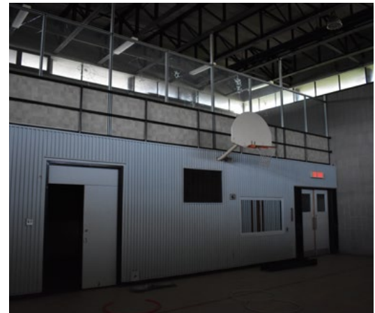
Figure 17. Building D, view of mezzanine (ERA, 2021).
