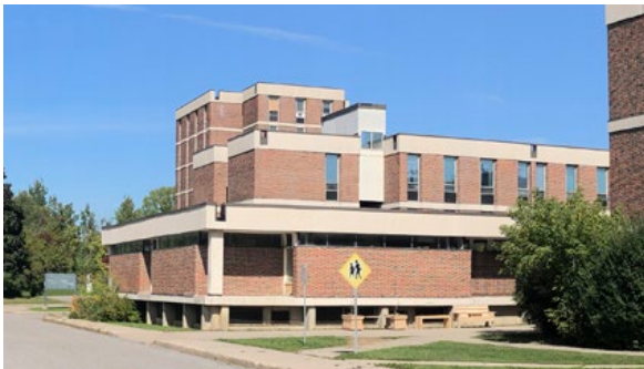
Building I, viewed from the southwest
