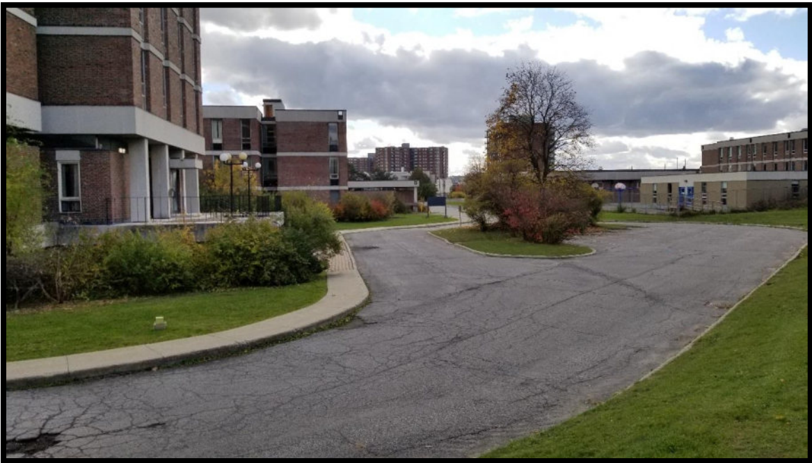
Photograph 3: View of the western portion of the Site, including Buildings K, J, and I (left to right, facing south).
