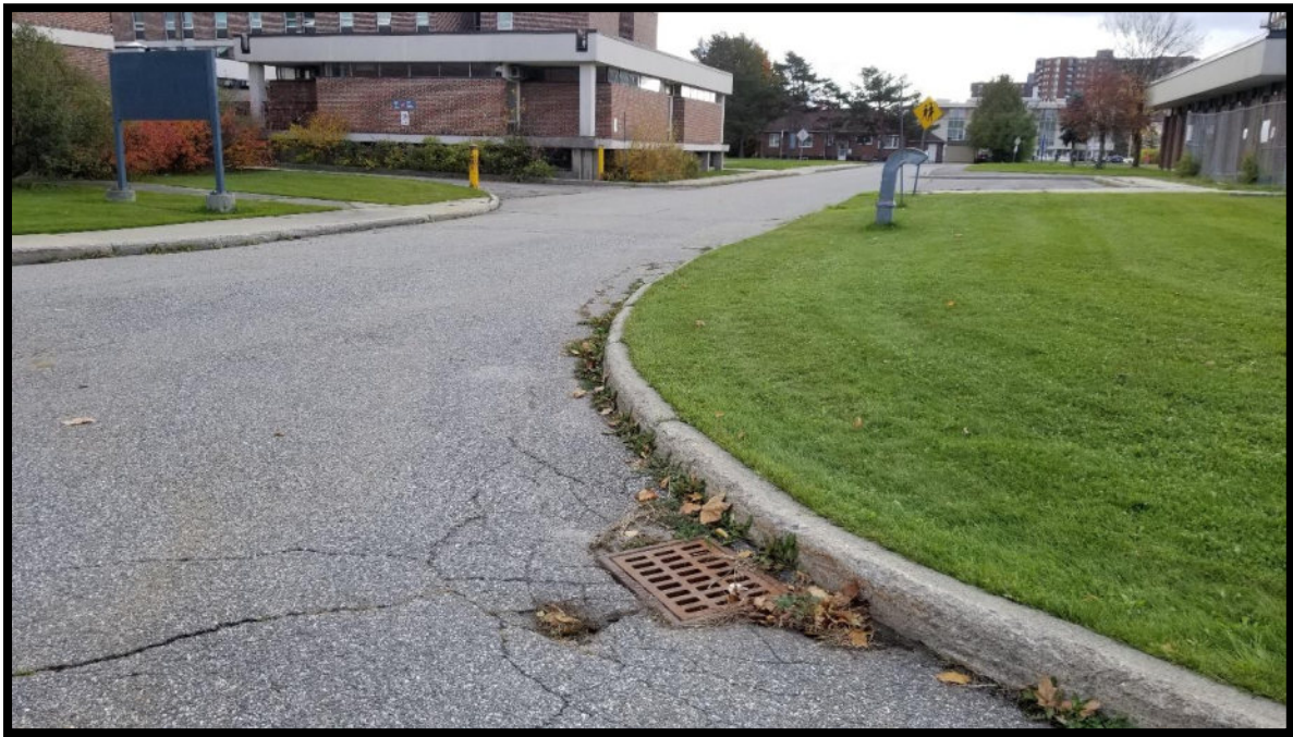
Photograph 13: View of the western edge of the complex, facing north.
