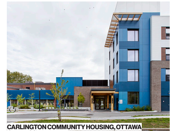
CARLINGTON COMMUNITY HOUSING, OTTAWA Source: GSV Architects
