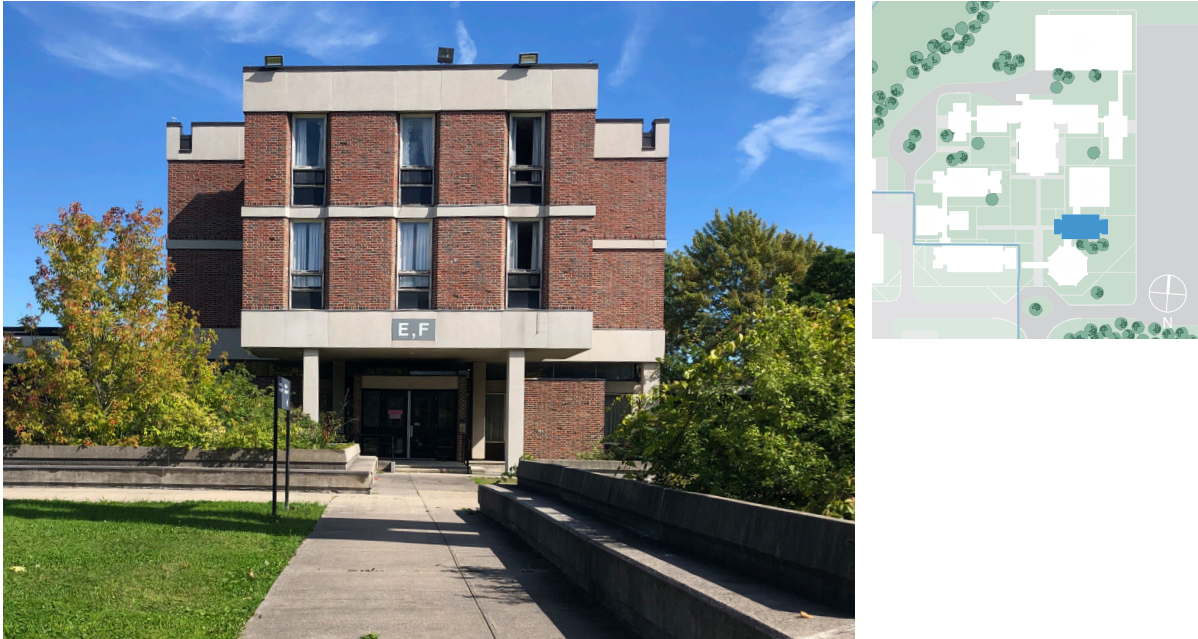
Figure 6. Building E, west elevation (ERA, 2021).
