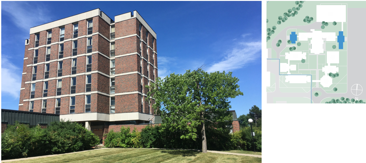
Figure 4. Building C, from novitiate courtyard (ERA, 2021).
