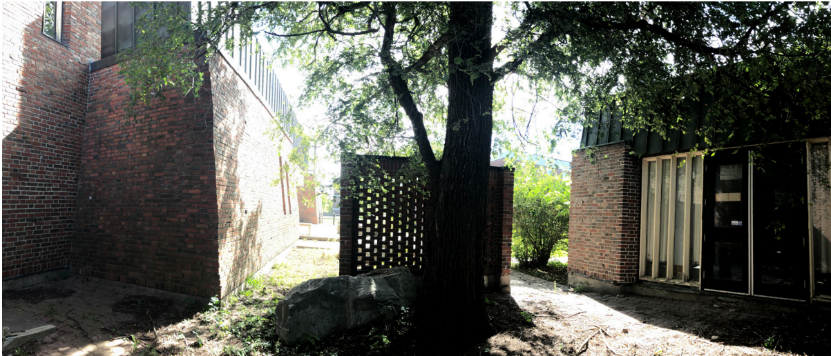
Figure 27. View from niche between Buildings A & L, looking toward the Sisters' Courtyard (ERA, 2021).
