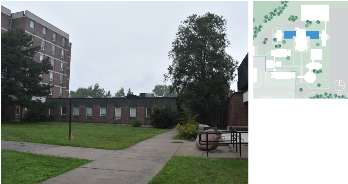
Figure 3. Building B, from Sisters' courtyard (ERA, 2021).
