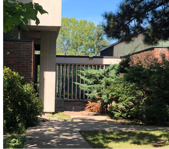
Figure 26. Niche at glazed link between Buildings K & L (ERA, 2021).
