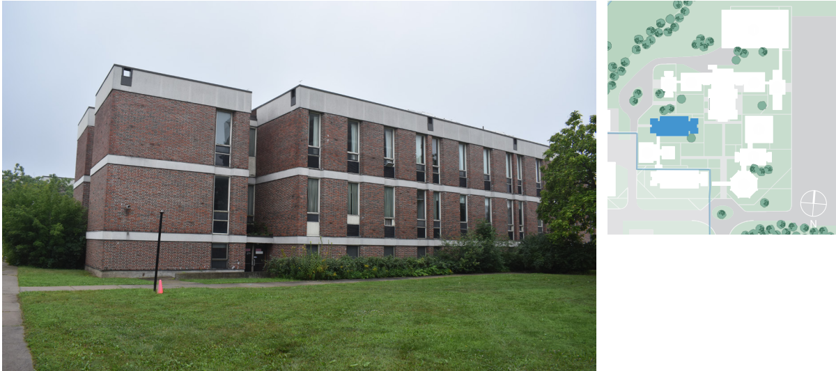
Figure 9. Building J, from Sisters' courtyard (ERA, 2021).
