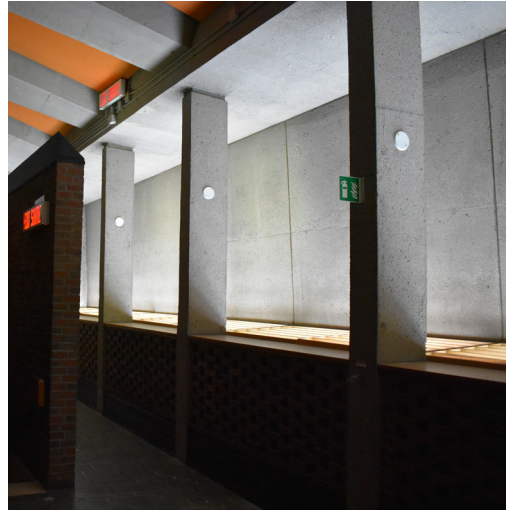
Figure 18. Building A, columns and water detail (ERA, 2021).
