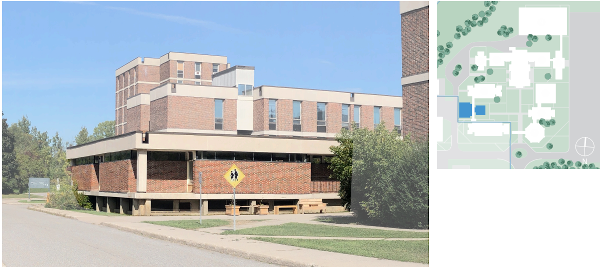
Figure 8. Building I viewed from southwest (ERA, 2021).
