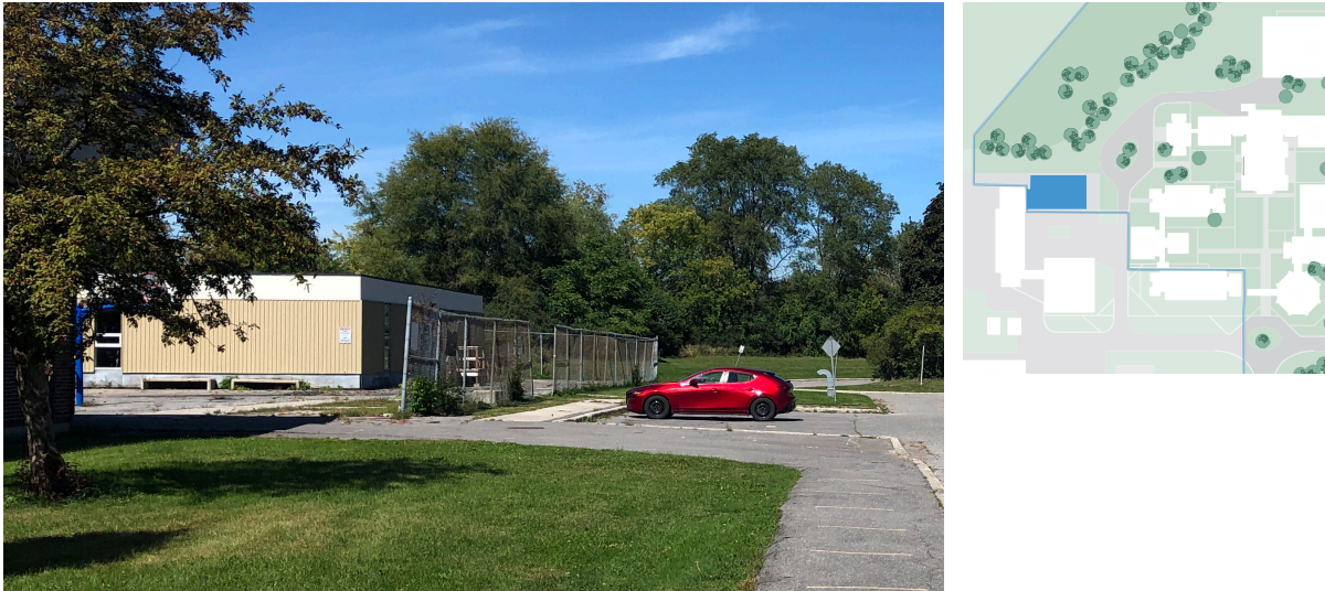
Figure 11. Building N, viewed from south-east (ERA, 2021).
