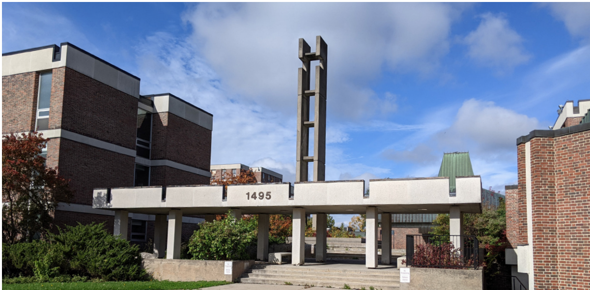
Figure 12. Main entrance canopy, with Campanile behind (ERA, 2021).
