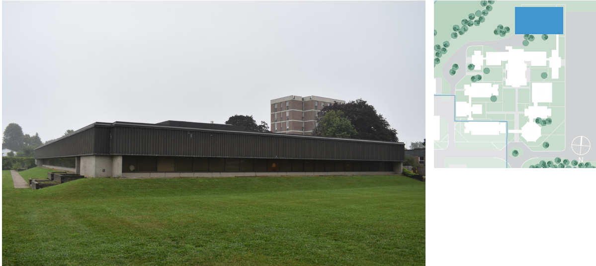
Figure 10. Building M, west elevation (ERA, 2021).
