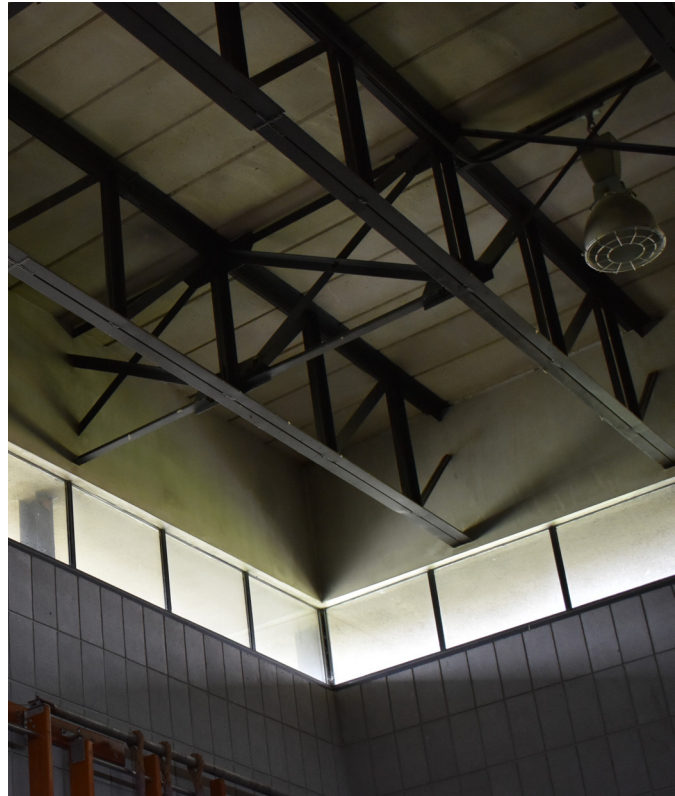
Figure 16. Building D, open web steel joist roof structure (ERA, 2021).
