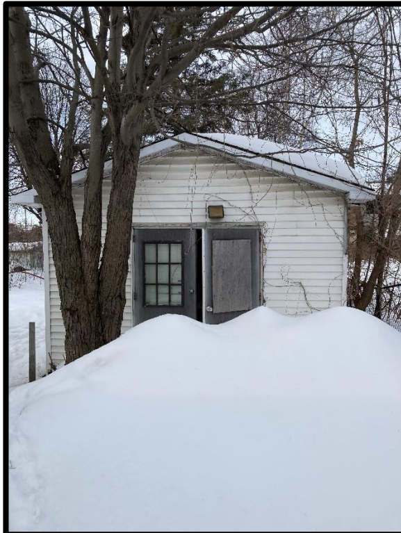
Photograph 6: View of the outbuilding on the 1196 Cummings Avenue property, facing west.
