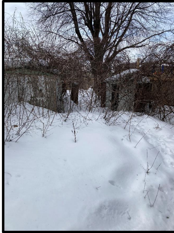
Photograph 7: View of the storage sheds on the 1196 Cummings Avenue property, facing south.
