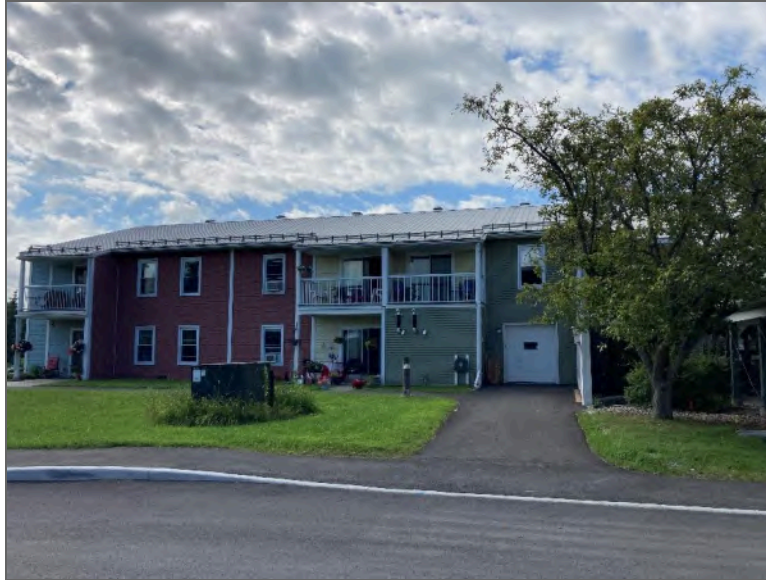
Photo 1 – Site Building (north elevation).
