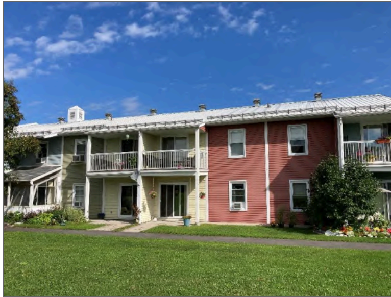
Photo 3 – Site Building (south elevation).
