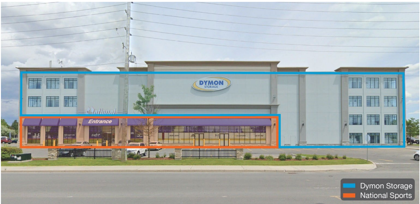
Figure 3: Street view of the subject property looking east on Lanthier Drive, with wall area color overlay.
