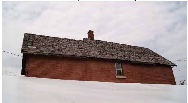
Roof (view from south)
