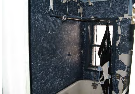
Second floor (bathroom)
