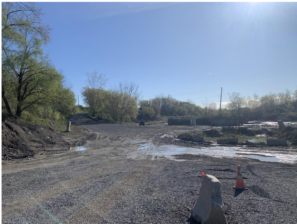
Photograph 4 – View of site facing east.
