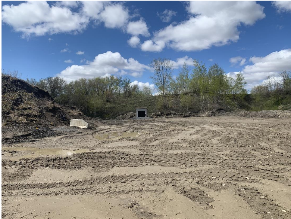
Photograph 7 - View site facing southwest
