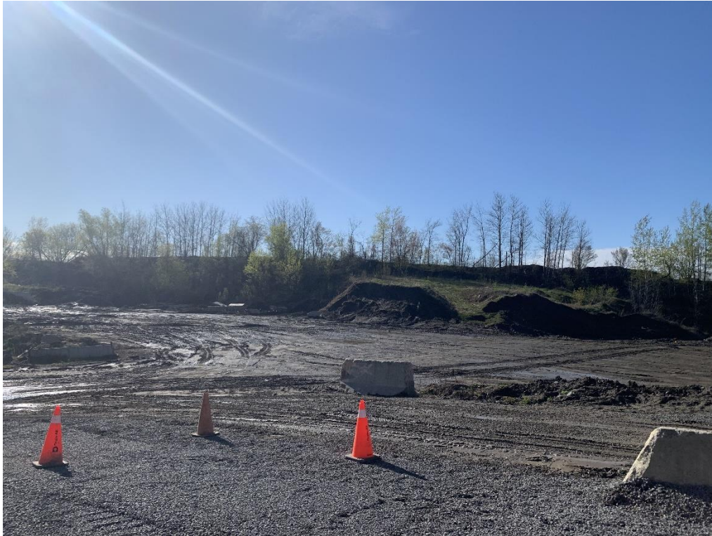
Photograph 5 - View of site facing east
