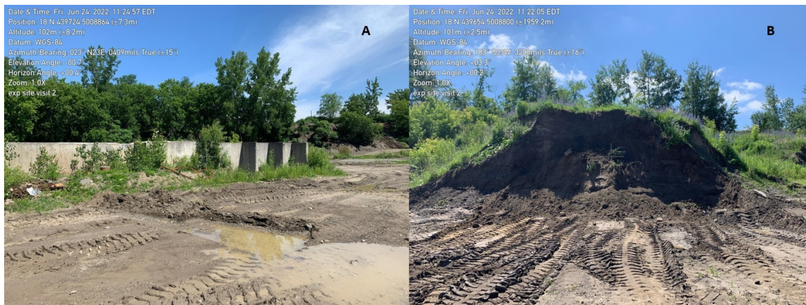
Figure 1 Photographs of the concrete structure in the center of the Site (A) and of a sandbank in the pit (B).
