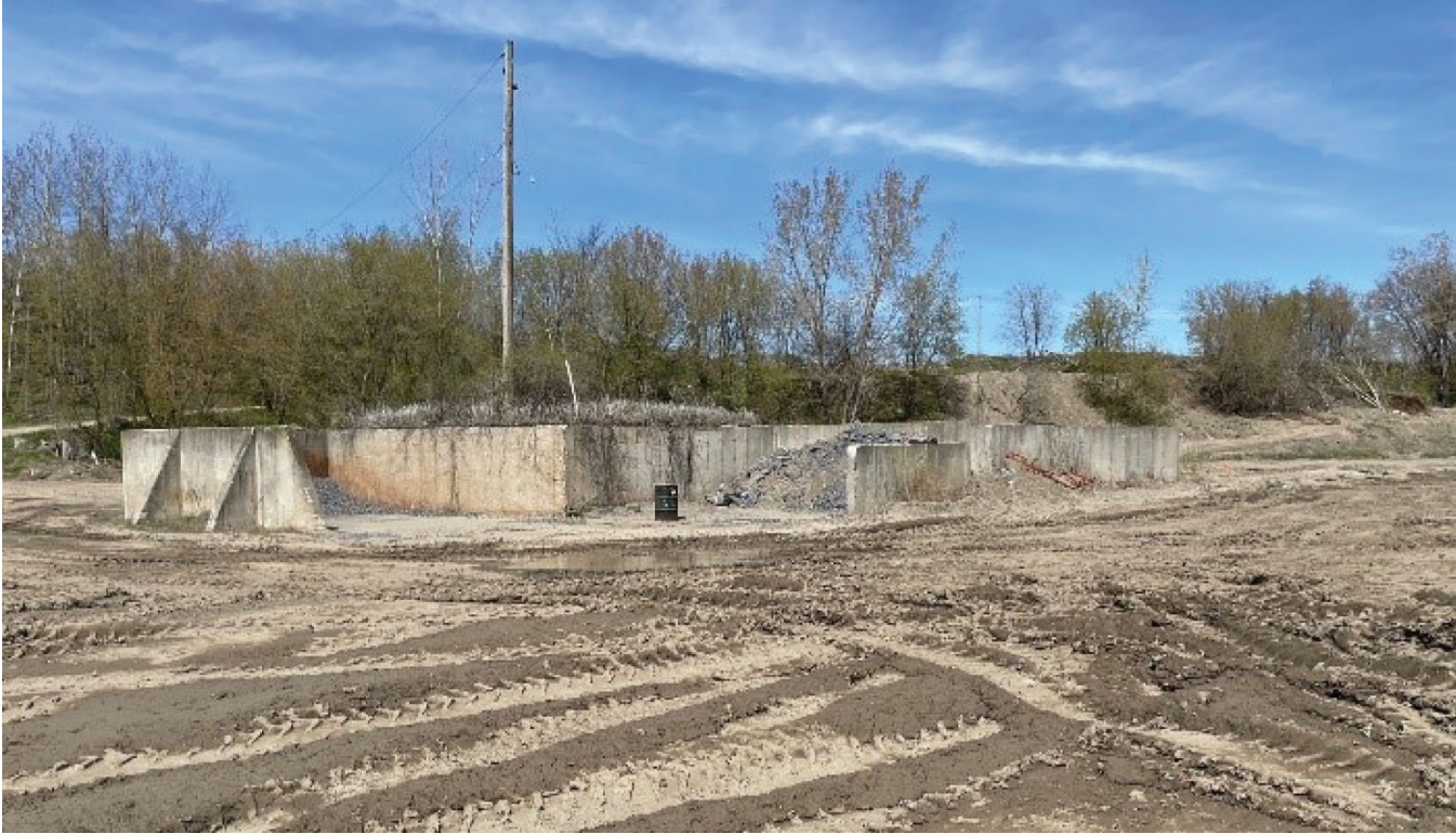
Figure 7: Image of concrete structure at the centre of the site, containing aggregates and overgrown vegetation.
