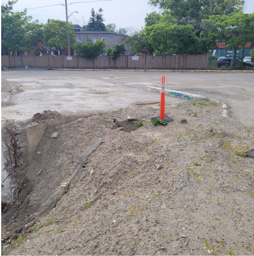
Photograph 5: View of the existing Waste Oil UST, which was emptied and had its contents disposed of off-Site in October 2022.
