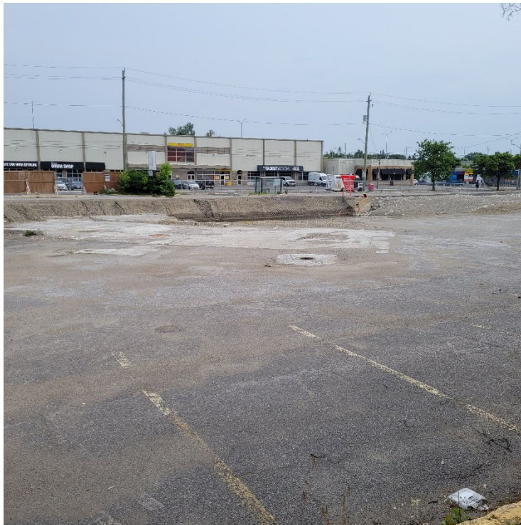
Photograph 4: View of the fill caps for the diesel UST and septic holding tank on the northeast portion of the Site. View is looking south.
