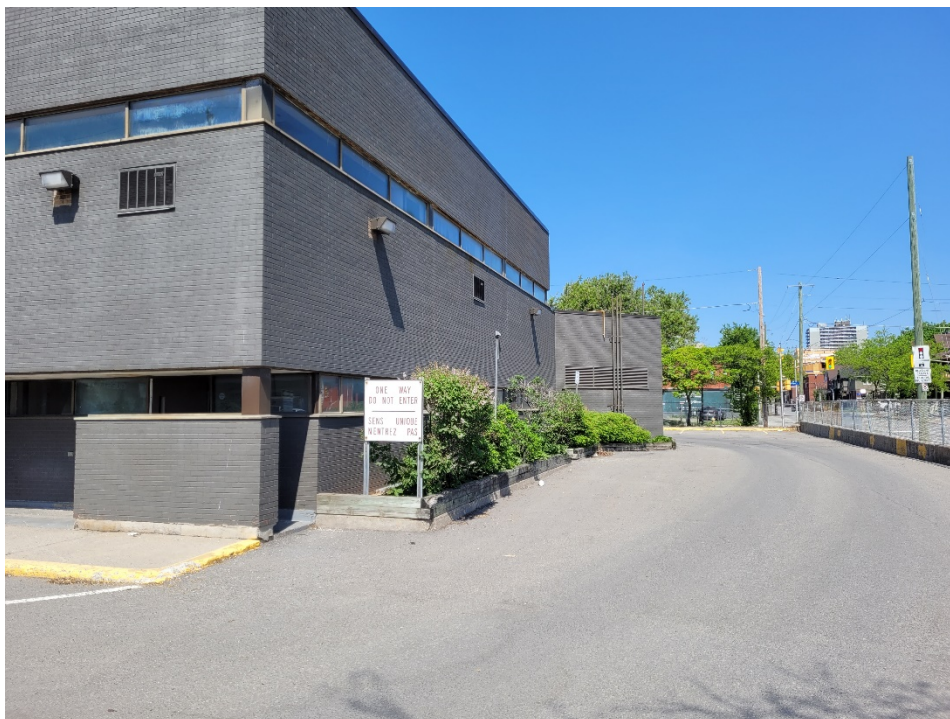
Photograph 2: View of Phase One Property looking north from the southeast corner of the Property. View shows the vent pipes associate with a former aboveground fuel storage tank and an underground waste oil storage tank, associated with the service garage on the east portion of the Property.
