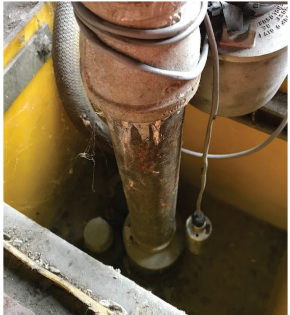
SENSOR LOCATED BENEATH DISPENSER
