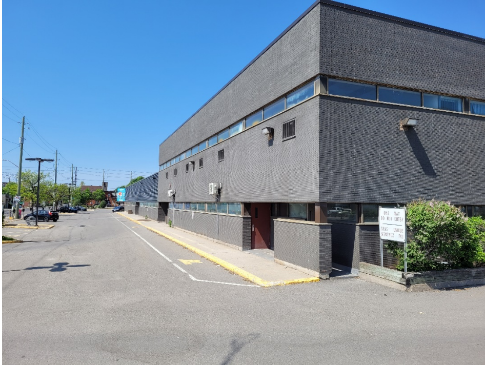
Photograph 1: View of Phase One Property looking west on the southeast portion of the Property. View shows the south side (front) of the commercial building at the Property.
