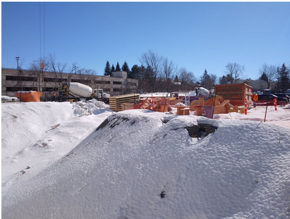
Photograph 4: View of the land immediately south of the Phase One Property, which is used as a construction staging area. The soil immediately adjacent to the south side of the building has been excavated and this area will provide access to the underground parking garage.
