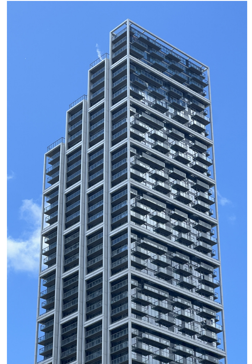
6000 MCKAY AVENUE, BURNABY, BRITISH COLUMBIA, CANADA
