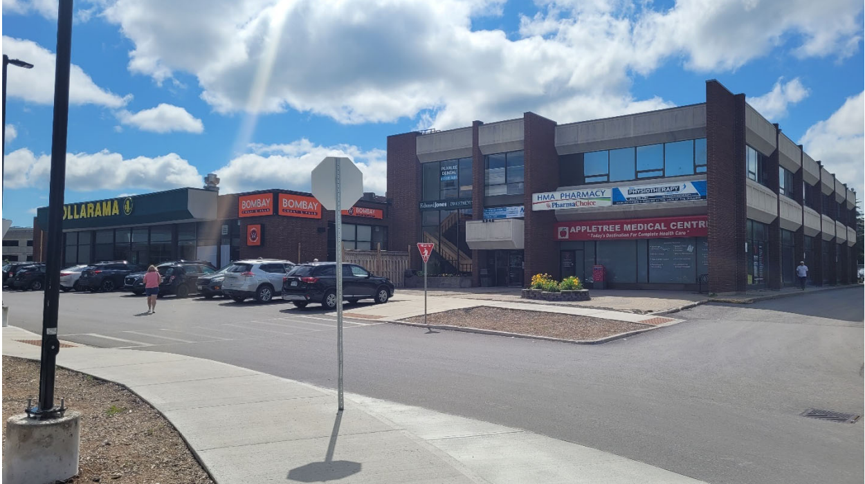
Photograph 1: View of north side of the Site building at the central portion of the Phase One Property looking south from south from the north parking area. View shows shared access road to the adjacent property to the east (also under Brigil ownership).
