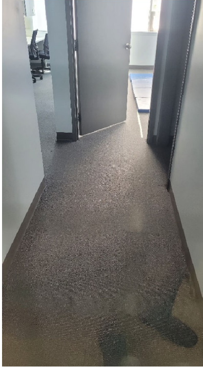
Photograph 5: View of the interior of a typical office space on the second floor of the Site building.
