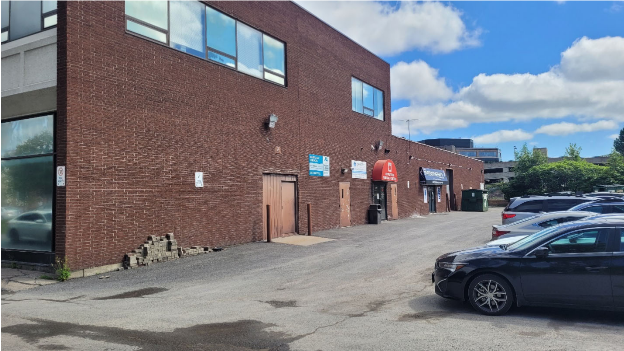
Photograph 2: View of north side of the Site building at the central portion of the Phase One Property looking east-northeast.
