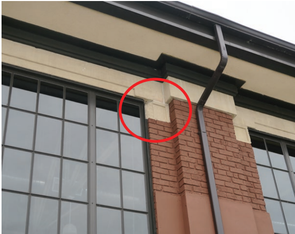
Chipped stone detail on east elevation (ERA 2023)
