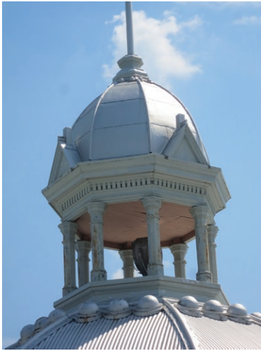
Dome roof cupola from north side (ERA 2019)
