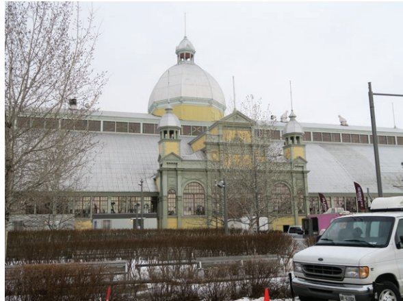
South elevation entrance pavilion (ERA 2023)
