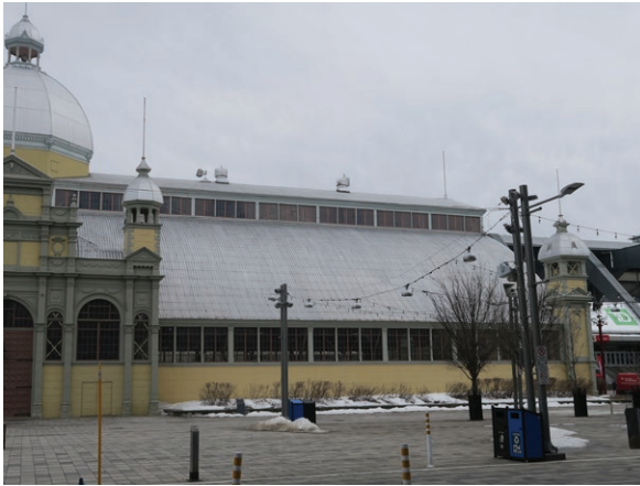
North upper roof: west section (ERA 2023)
