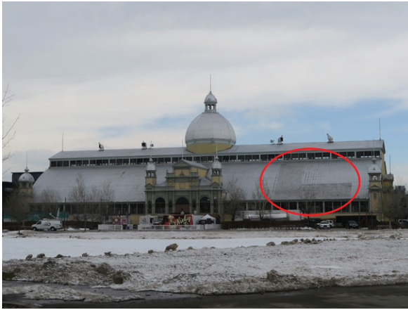
South lower roof. Note fabric covering (ERA 2023)
