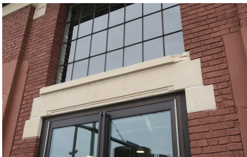
Chipped stone sill above door on east elevation of the exhibition hall (ERA 2023)
