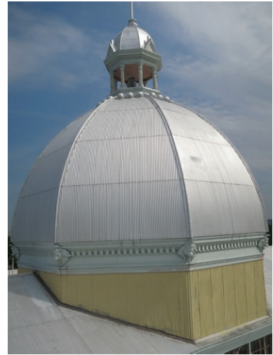
South view of roof dome (ERA 2019)
