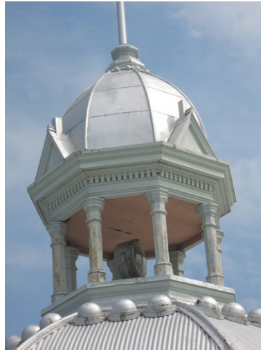
Roof cupola from south (ERA 2019)
