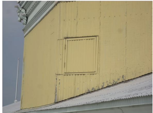
Base of roof dome from south side (ERA 2019)
