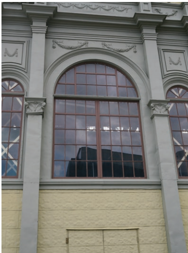
Entrance Pavilion window on north elevation (ERA 2023)
