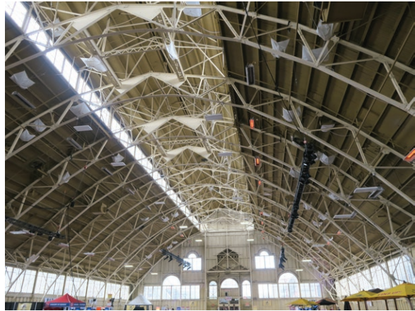
Interior underside of roof: looking west (ERA 2019)
