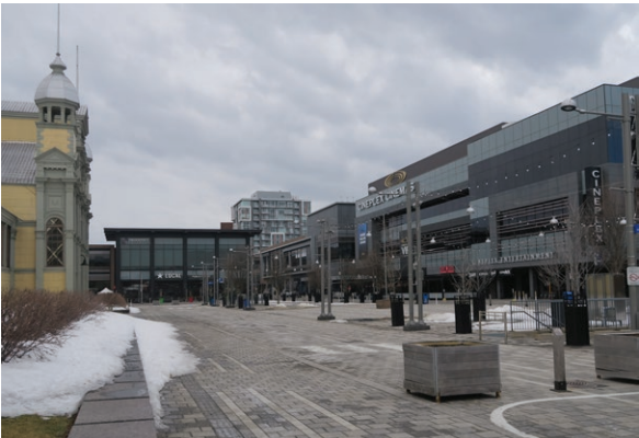
Looking west towards Aberdeen Square (ERA, 2023).
