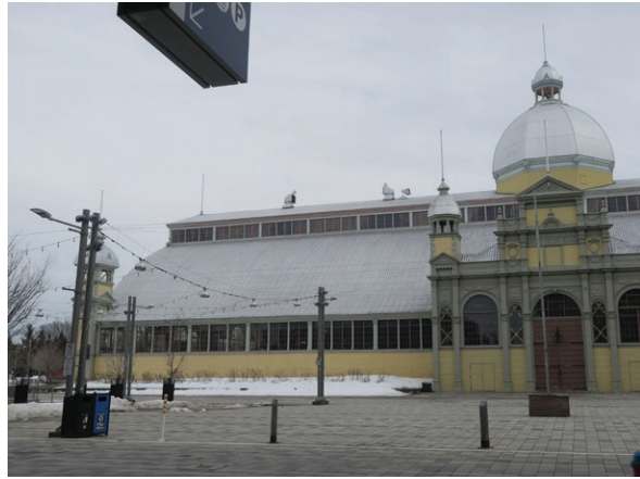
North upper roof: east section. (ERA 2023)
