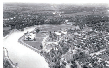
1927 aerial of the Rideau Canal looking south towards Lansdowne Park (National Resources Canada).
