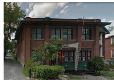
115-117 Holmwood Avenue (Google, 2016).
