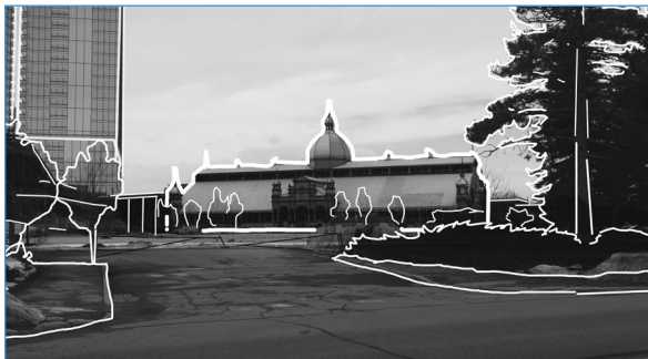
Three-Tower Concept: View from Queen Elizabeth Driveway toward the Site (ERA, June, 2023).
