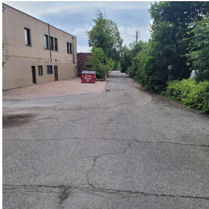
Photograph 2: View of the of the north portion of the Phase One Property looking west. View shows the 2-storey office building on the east portion of the Property.
