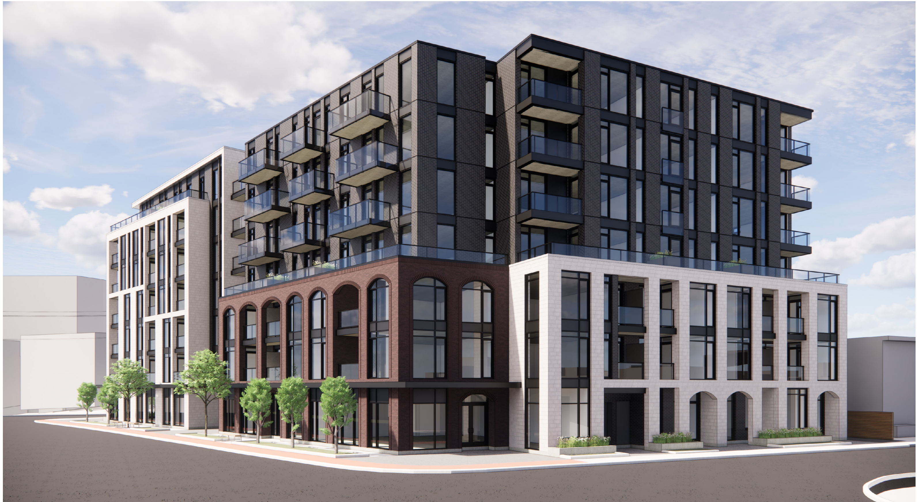
47 BEECHWOOD AVENUE VIEW FROM CORNER OF BEECHWOOD AND DOUGLAS
