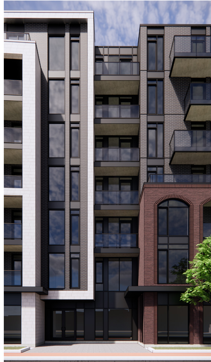
VIEW OF CENTER BREAK IN MASSING
