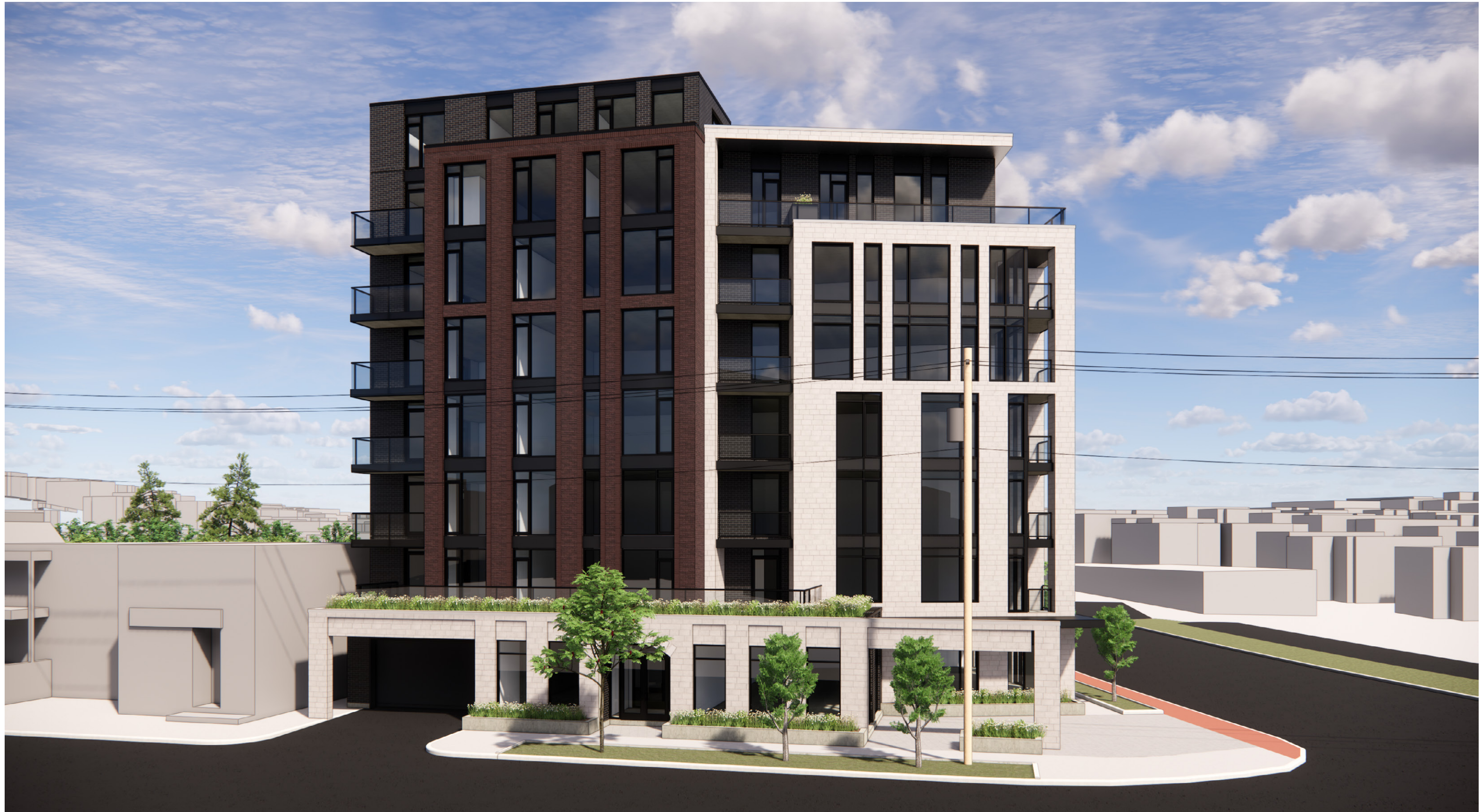
47 BEECHWOOD AVENUE VIEW OF SPRINGFIELD ELEVATION
