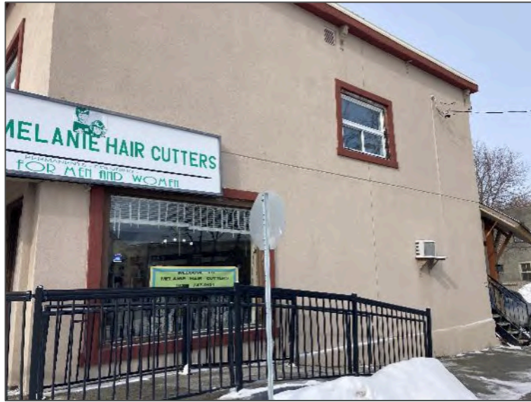
Photo 11 – East elevation of Site Building D, looking northwest.
