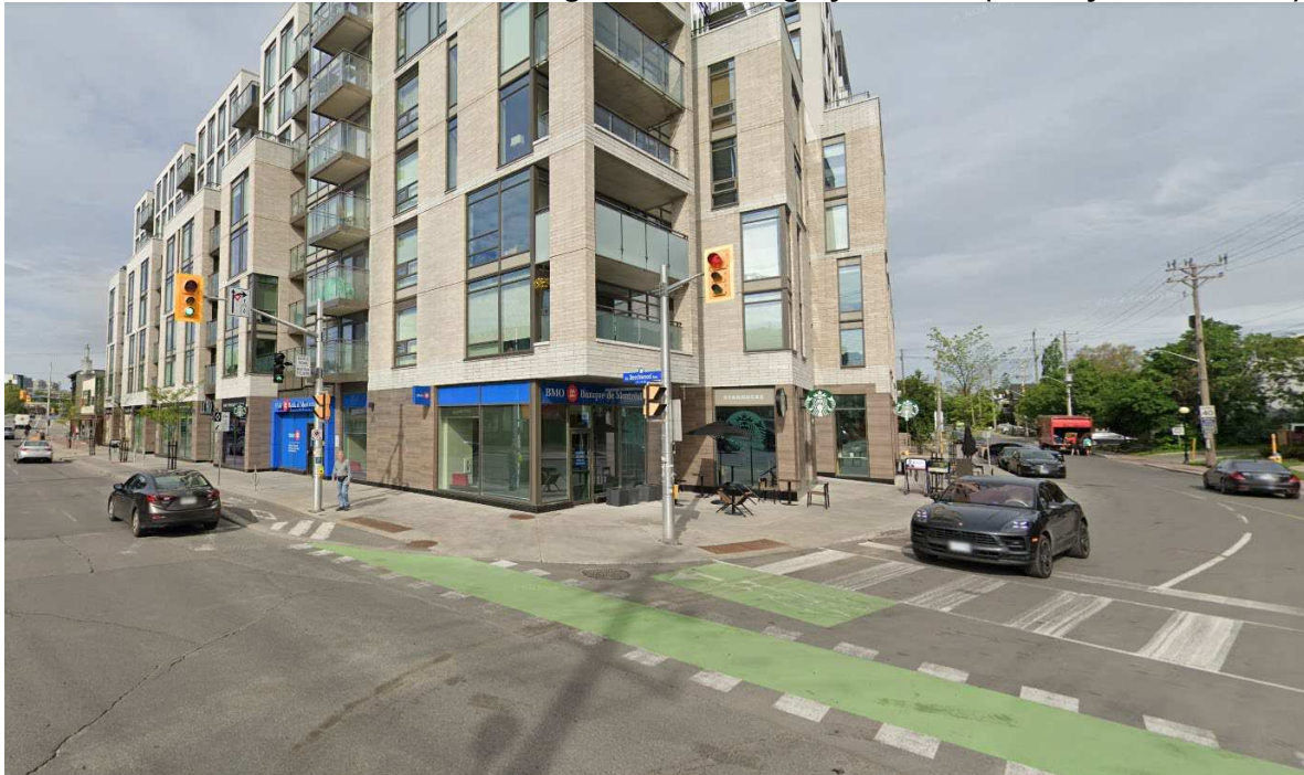
Figure 21: Existing Cycle Track (MacKay / Beechwood)
