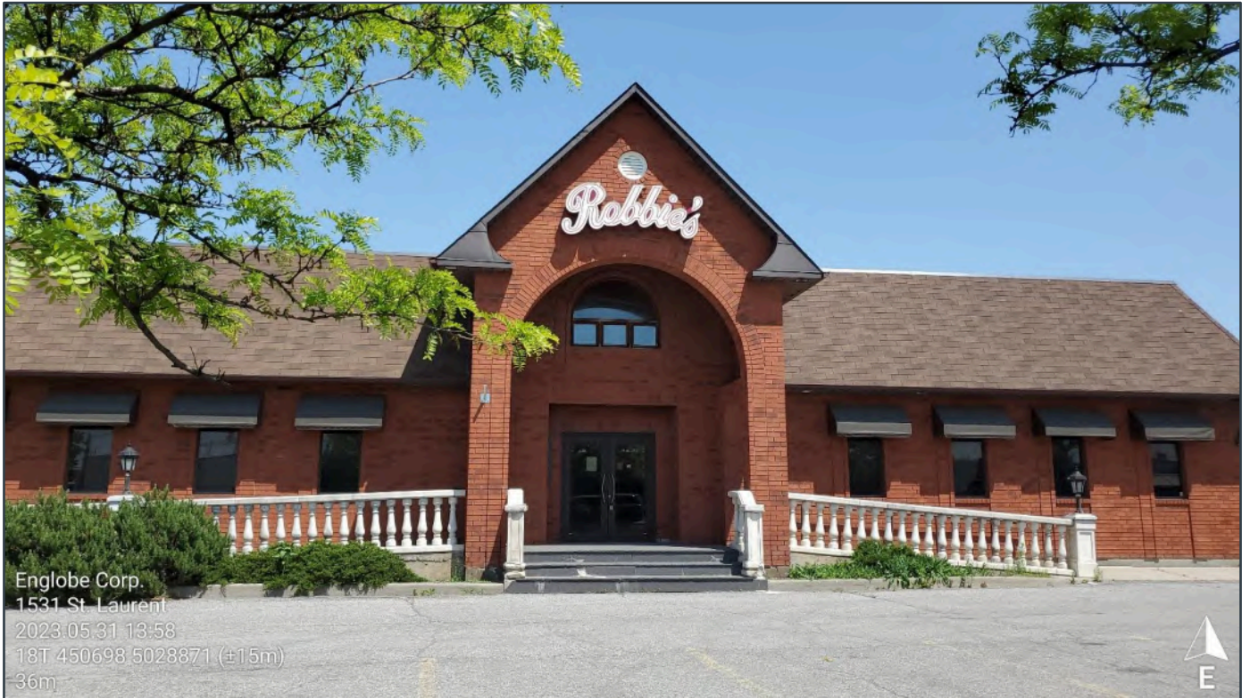
Site Photograph 1: Overview of the Site.
