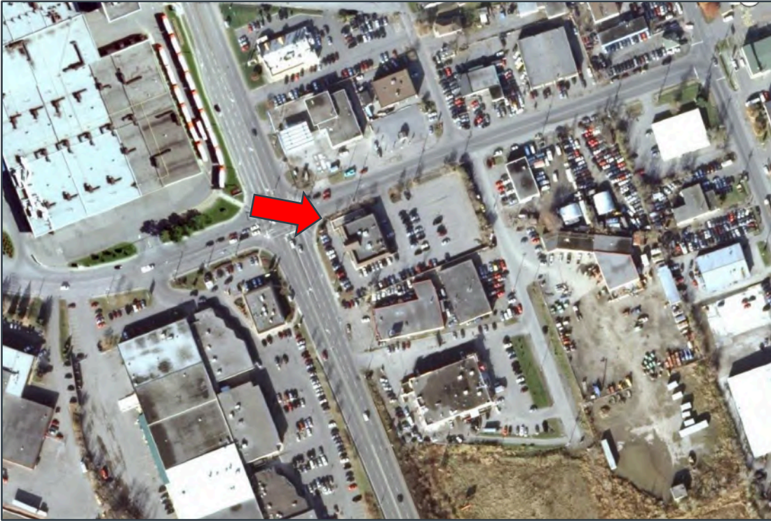
City of Ottawa Aerial Photograph (2011)
