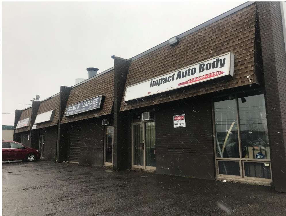
Photo 7: Multiple automotive service stations located to the northeast of the Site.
