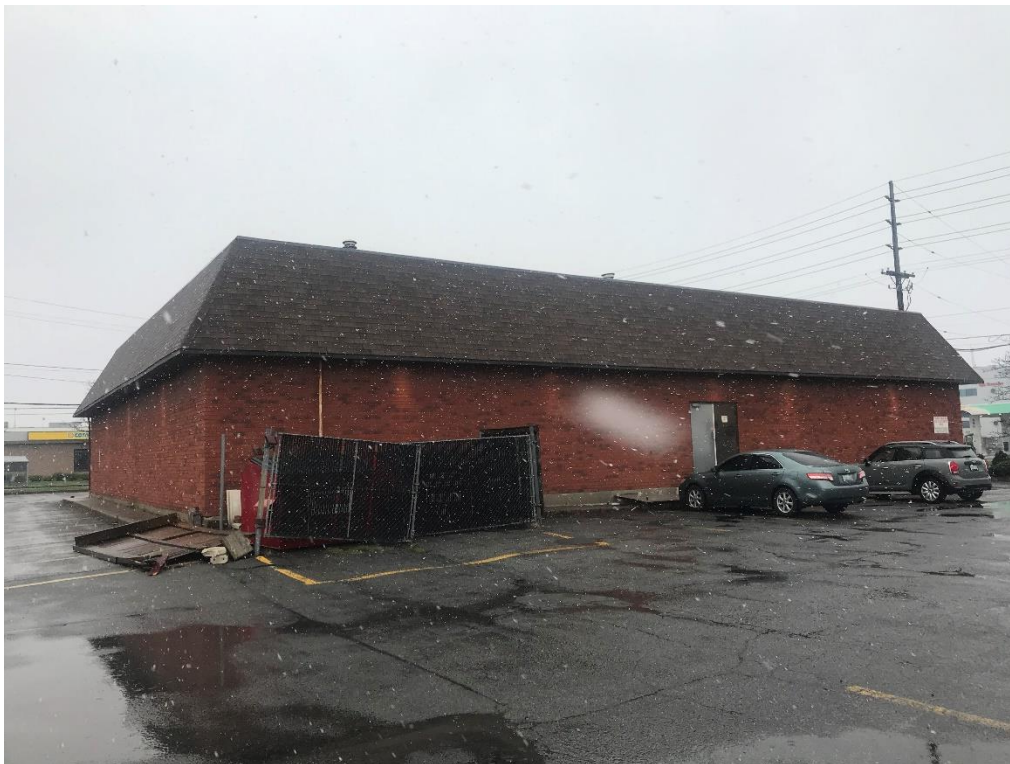
Photo 2: Eastern elevation of the Site building, facing west.
