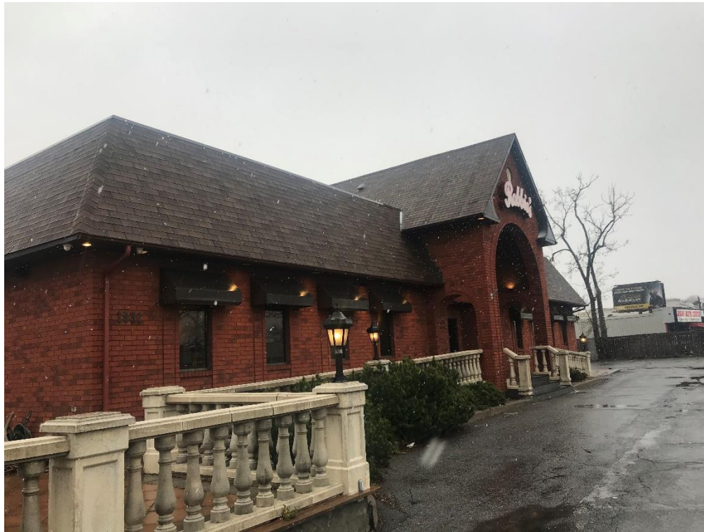
Photo 1: Western elevation of the Site building, facing south.
