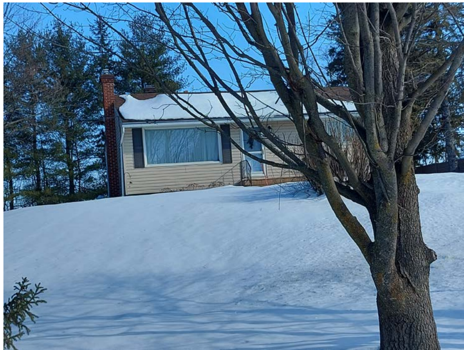
View of residential dwelling located south of site
