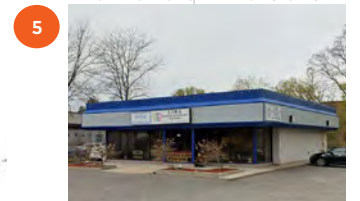
797 RICHMOND RD. EXISTING 1-STORY DENTAL OFFICE
