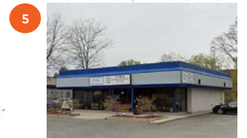
797 RICHMOND RD. EXISTING 1-STORY DENTAL OFFICE
