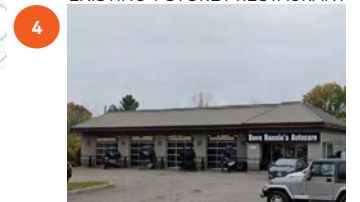
801 RICHMOND RD. EXISTING 1-STORY AUTO SHOP
