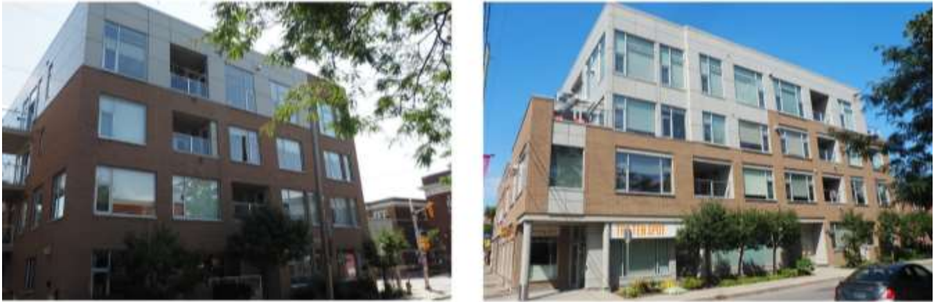
Figure 6: North (left) and south (right) building faces.
